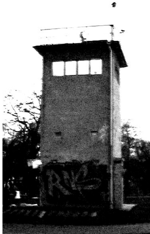
FOTO 1: Watch tower at former Berlin Wall
