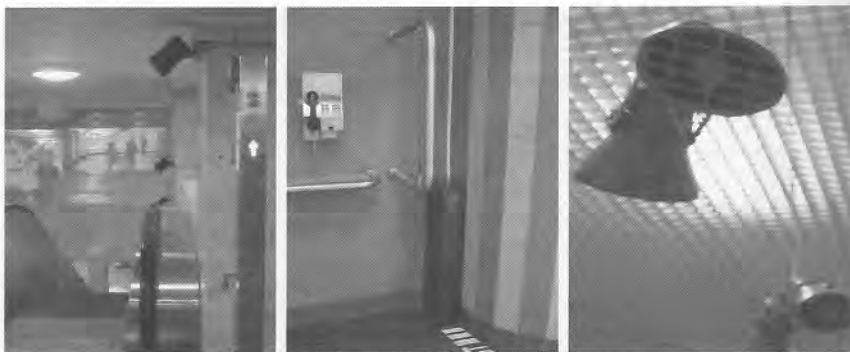
Figure 23: Loudspeaker-pairs in Warsaw whose front grilles corresponded to the structure of the ceiling.
